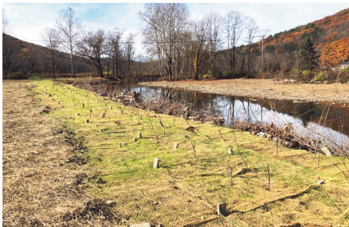
Root wad armoring, willow staking, and seed matting along Oquaga Creek as part of a stream restoration project with Trout Unlimited, located in the Delaware River Watershed, NY.
